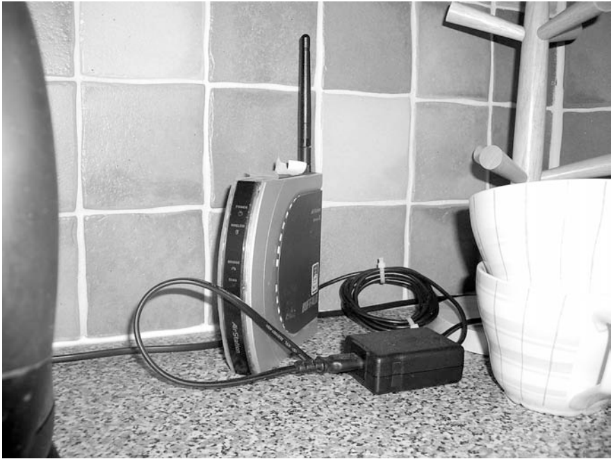
Figure 4.2 “AirStation” in the kitchen.
